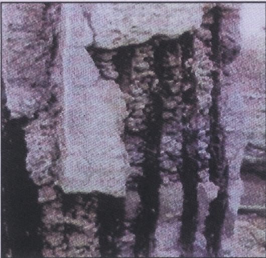
C2 - Severe Column reinforcement corrosion
