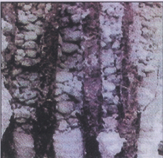
C2 - Severe Column reinforcement corrosion
